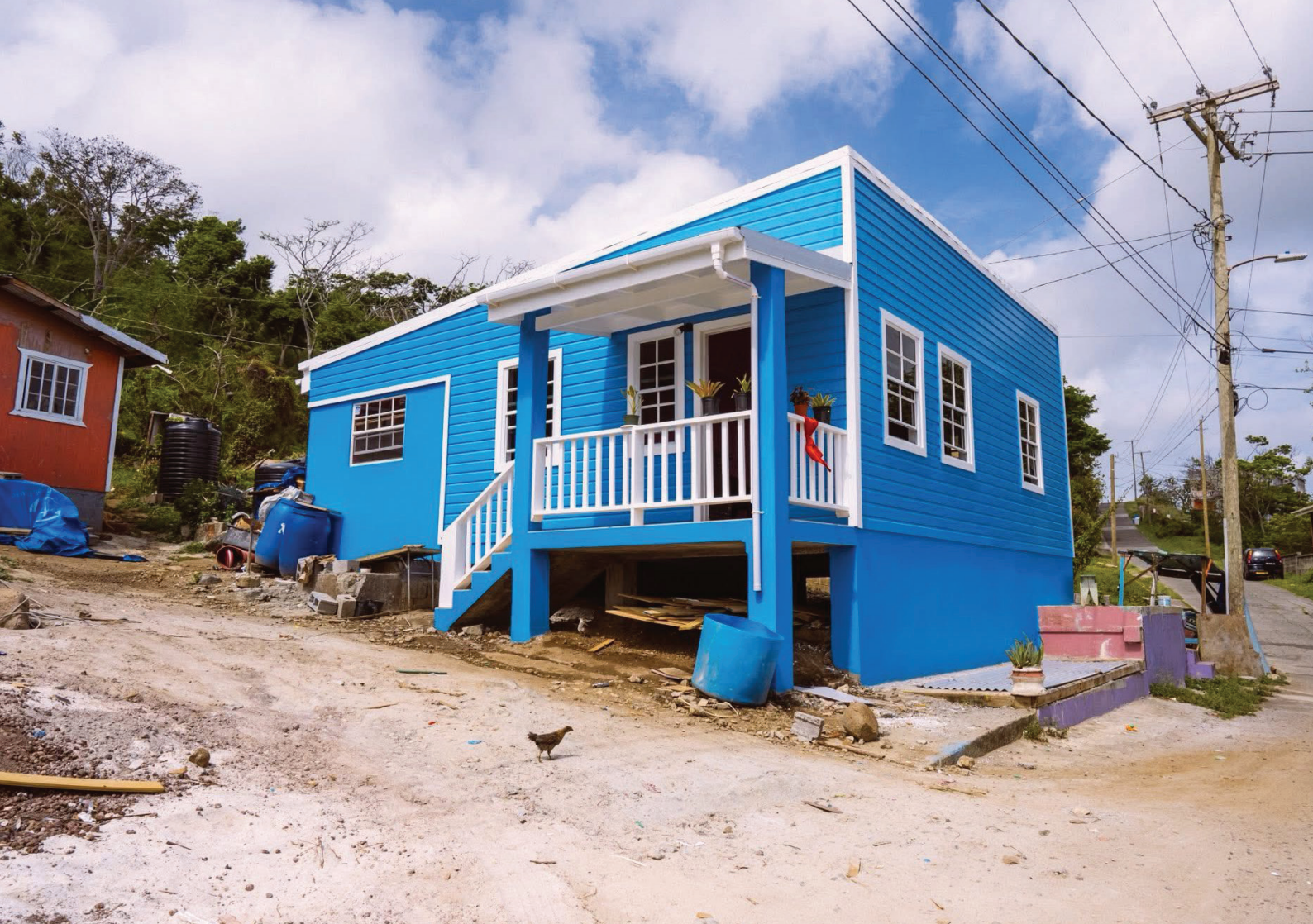
100 low-income housing units in Dumfries, Carriacou
