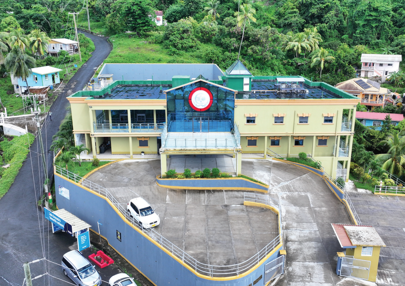
Gouyave Health Centre, St. John
