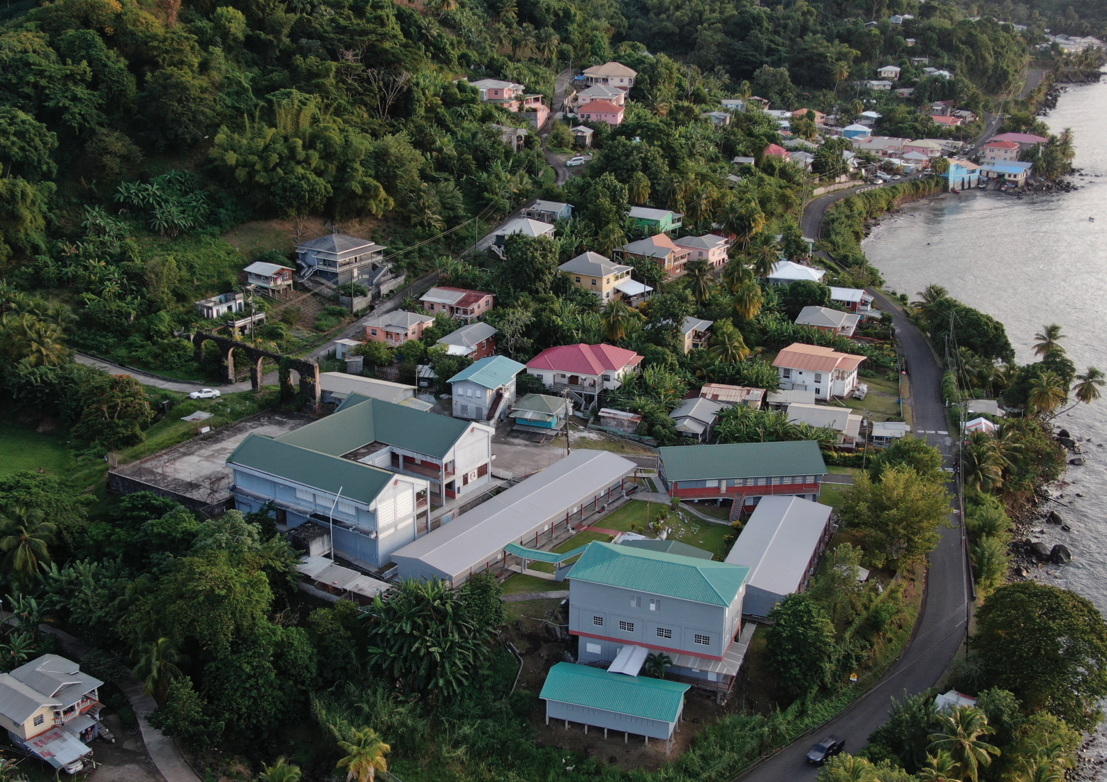
Exterior of the newly rebuilt St. Mark's Secondary School, showcasing climate-smart infrastructure supported by the OECS Human Mobility Project
